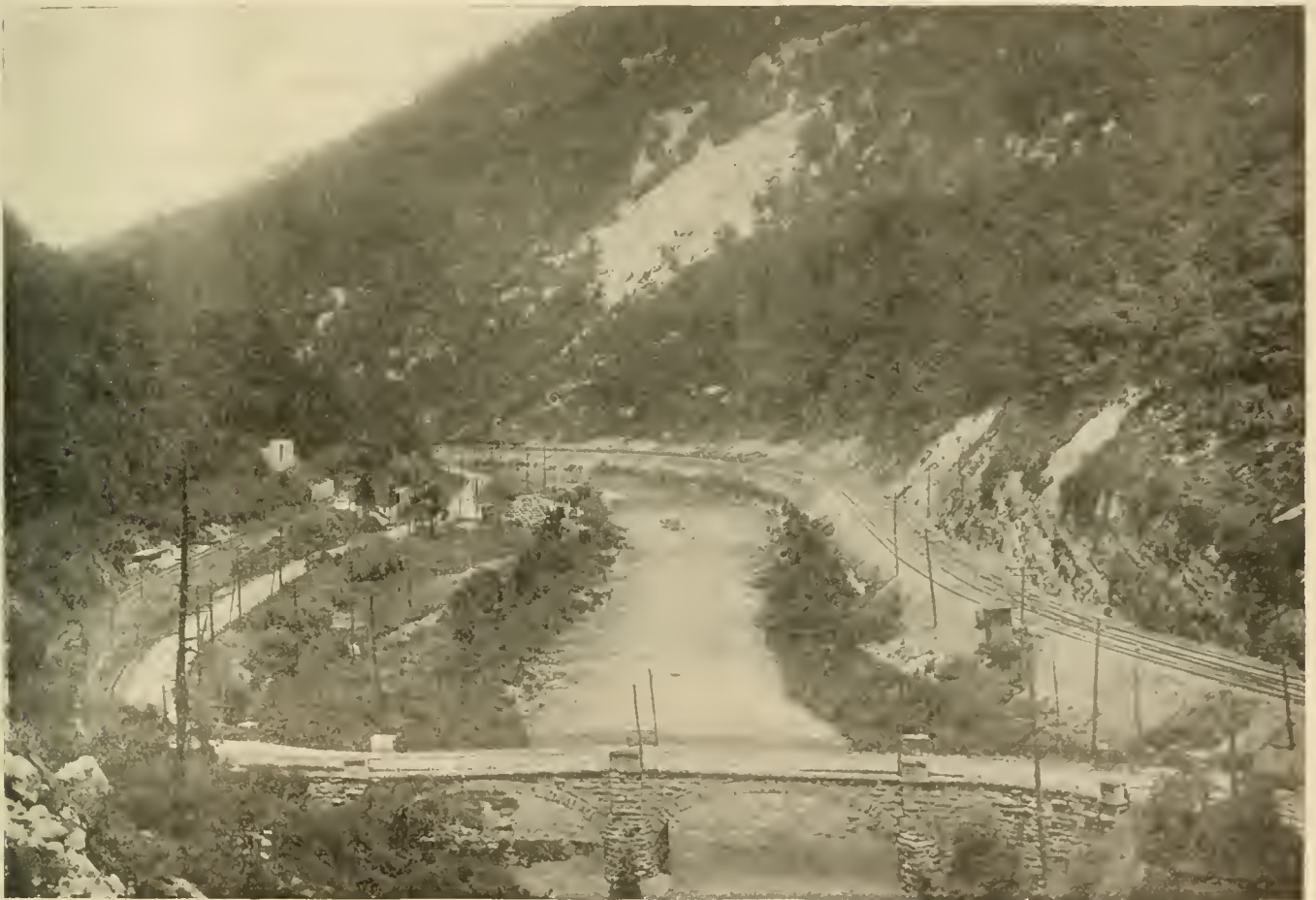
CUMBERLAND NOTCH IN MARYLAND, SHOWING NATIONAL HIGHWAY AND TWO LINES OF RAILROADS.
